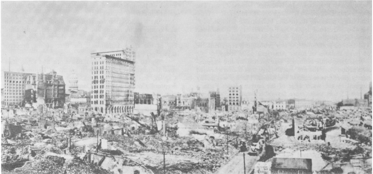
Figure 20.—Baltimore after the fire, looking down Lombard Street. Brick buildings crumbled. Fireproof buildings were gutted. The Continental Trust Building is behind the large structure at left center. (Reproduced from Baltimore Afire , published and copyrighted by Schneidereith & Sons, Baltimore, Maryland.)
